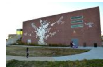
The Stream Rises Above the Fountain (2014.5.1)
