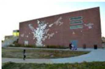
The Stream Rises Above the Fountain (2014.5.1)
