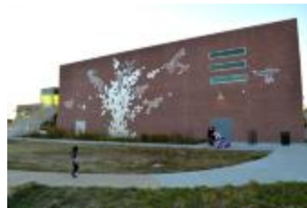
The Stream Rises Above the Fountain (2014.5.1)
