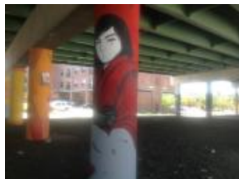
Evans Bridge Project (UAF.2018.15)
