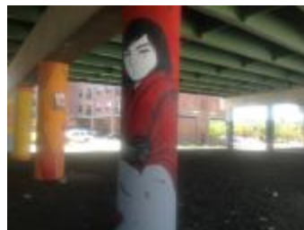
Evans Bridge Project (UAF.2018.15)
