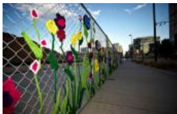
Central Platte Construction Fence (2010.12.2)
