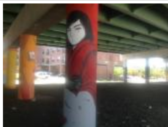
Evans Bridge Project (UAF.2018.15)
