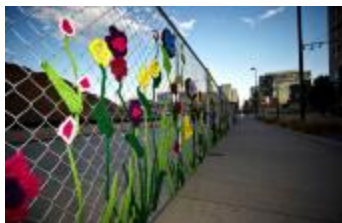
Central Platte Construction Fence (2010.12.2)
