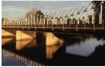
Bridge of Recycling Fountains (1996.1.1)
