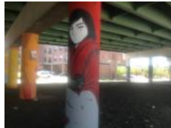
Evans Bridge Project (UAF.2018.15)
