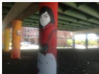
Evans Bridge Project (UAF.2018.15)
