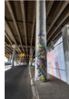
Untitled (colorful concrete columns painted under I-70) (UAF.2017.38)
