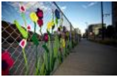
Central Platte Construction Fence (2010.12.2)
