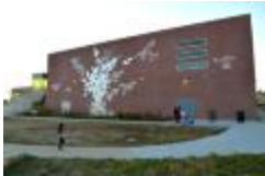
The Stream Rises Above the Fountain (2014.5.1)
