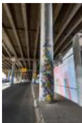
Untitled (colorful concrete columns painted under I-70) (UAF.2017.38)
