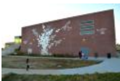
The Stream Rises Above the Fountain (2014.5.1)
