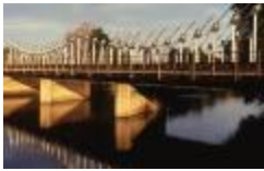
Bridge of Recycling Fountains (1996.1.1)
